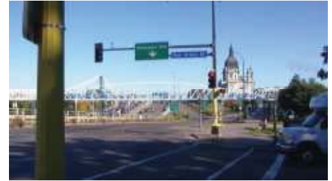
Hennepin-Lyndale Corridor, above western entry to Lowry Tunnel
