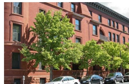
An historic apartment building with young street trees along 16th Street
