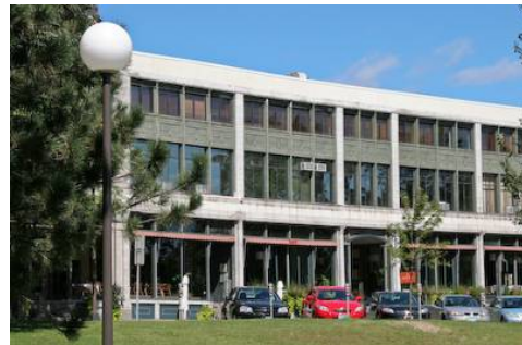
Parking along Harmon Place near the Fawkes Block
