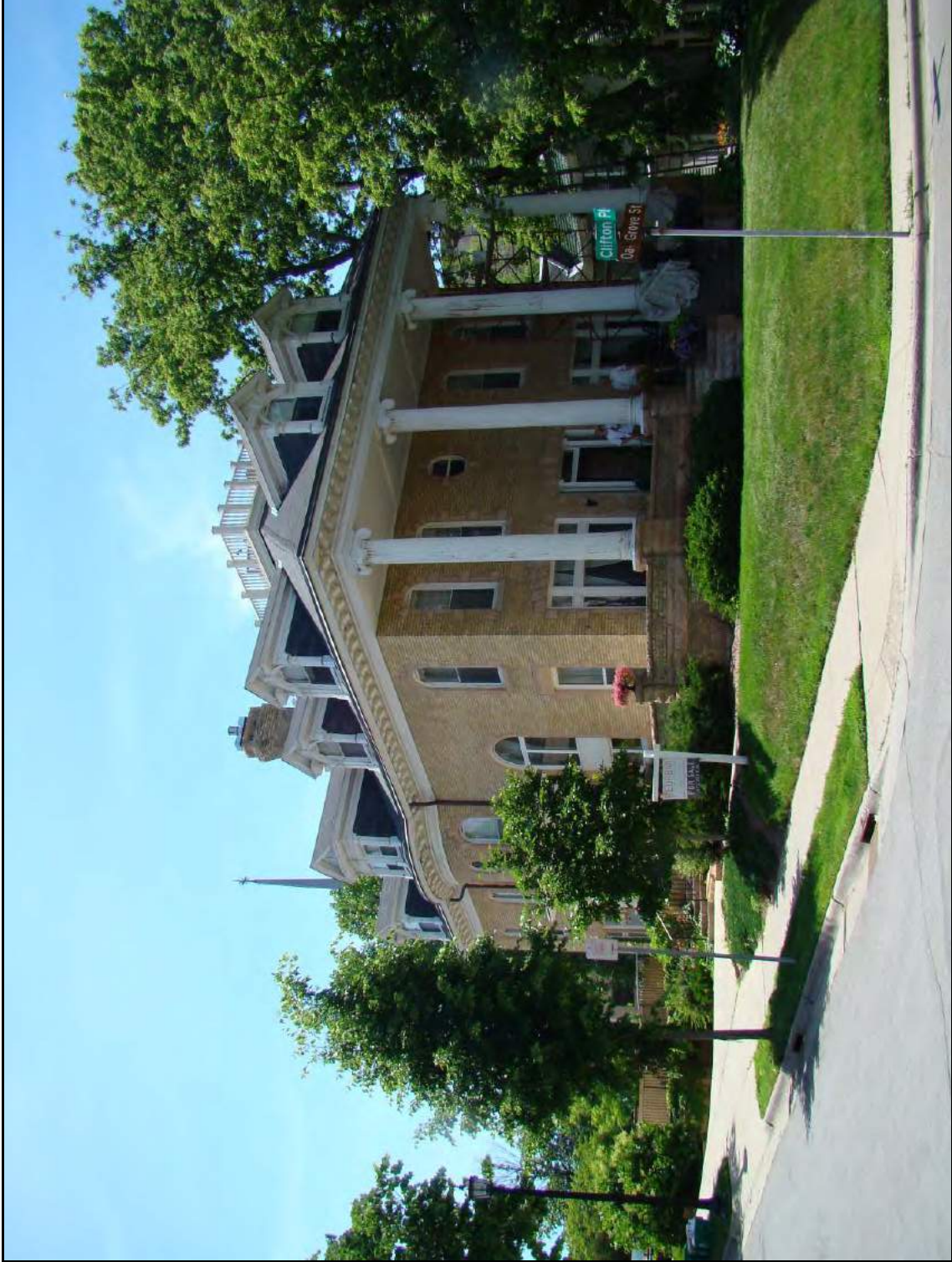
Figure 3: Daniel B. Lyon House- North and East Elevations, 2010, Source: CPED Files
