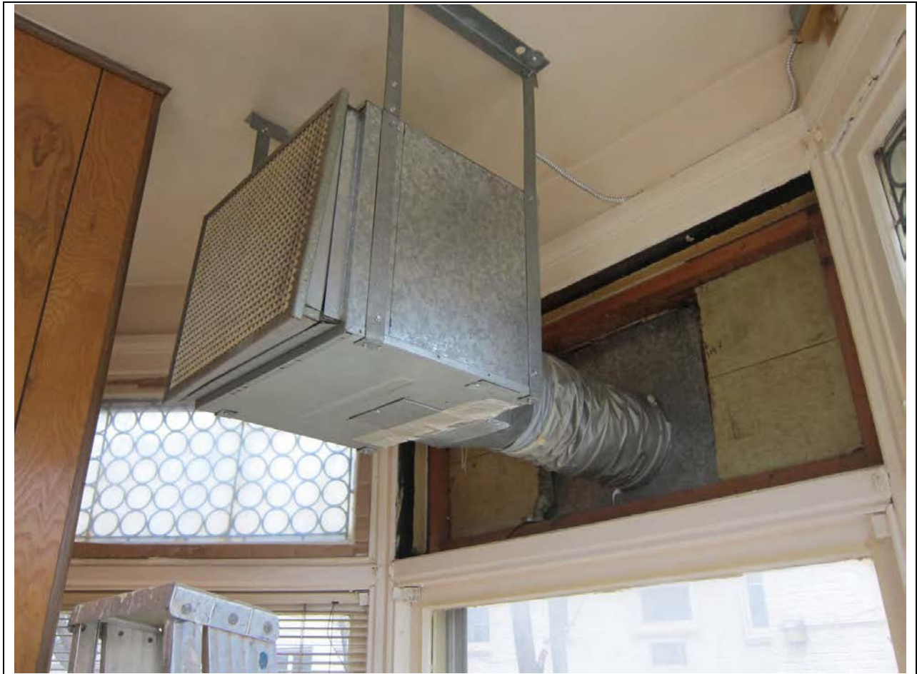
Figure 38. Nonhistoric fan box in turret, facing northeast, November 2010, source: CPED files
