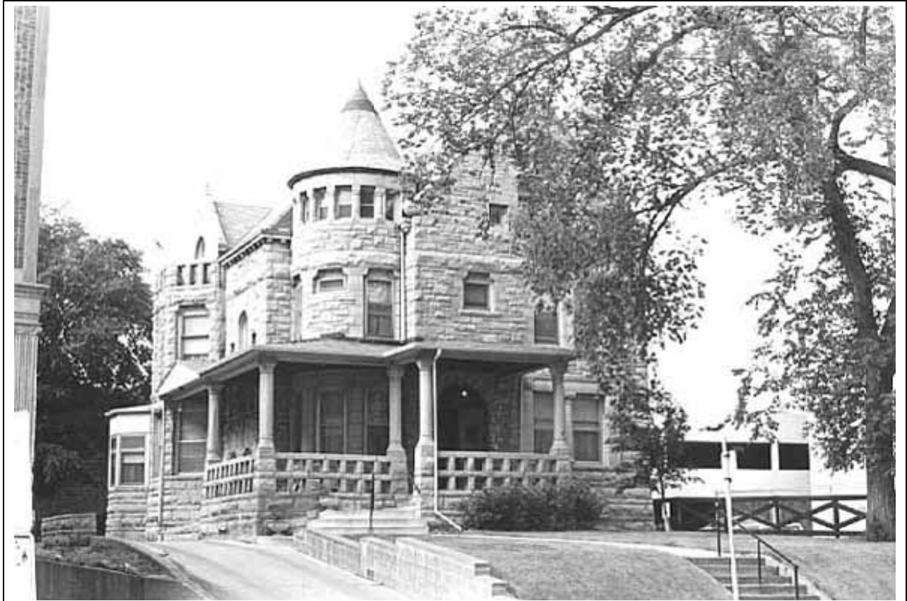
Figure 51. Ladd House, June 1974, two years after conversion of home to a care center, source: Minnesota Historical Society, note removed porte cochere on left side of porch
