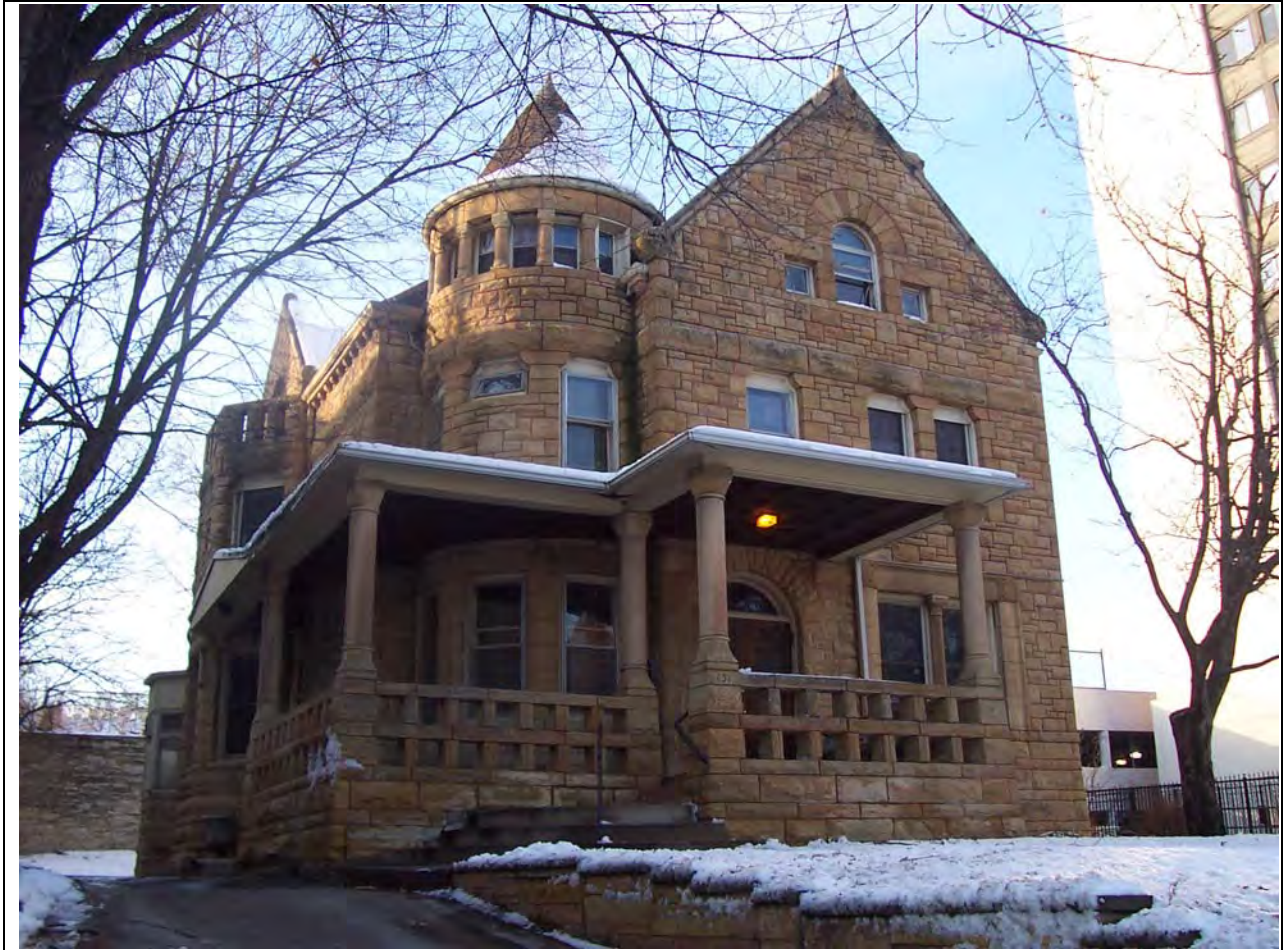
Figure 52. 131 Oak Grove Street, front (north) elevation and wraparound porch, looking southwest, November 2010, source: CPED files
