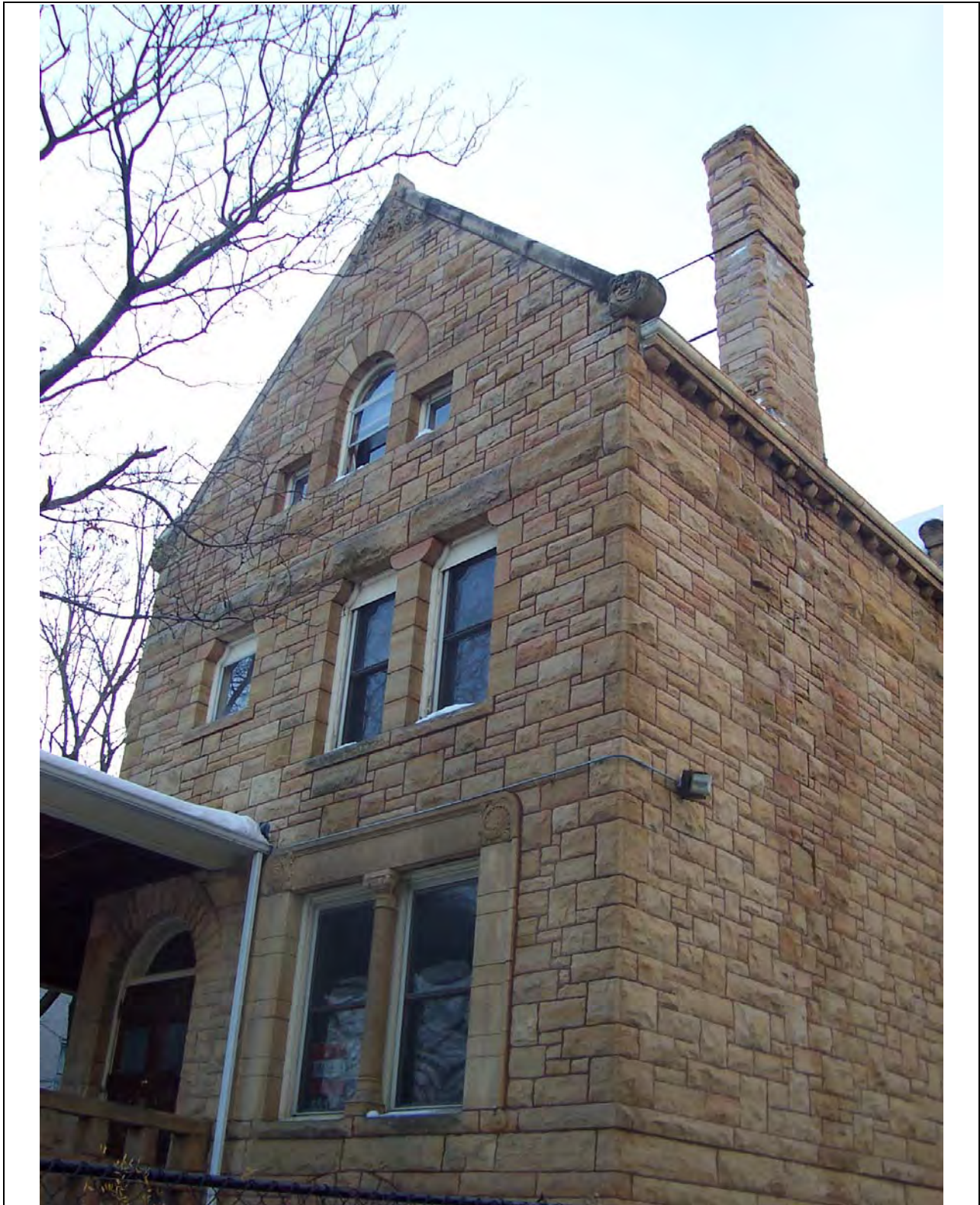
Figure 4. Chimney on northwest building corner, November 2010, source: CPED files
