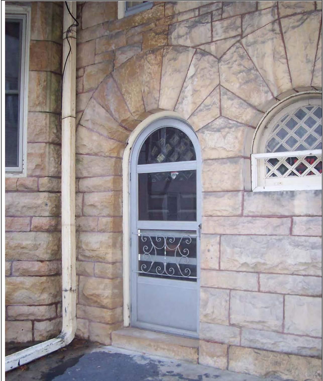
Figure 7. Side (east) entrance, looking west, November 2010, source: CPED files
