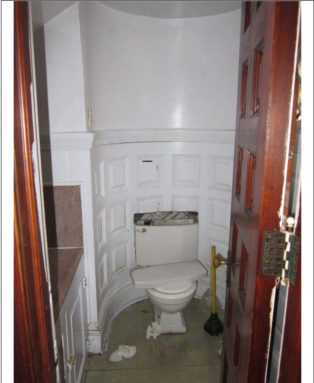
Figure 55. Entryway bathroom, facing north, November 2010, source: CPED files
