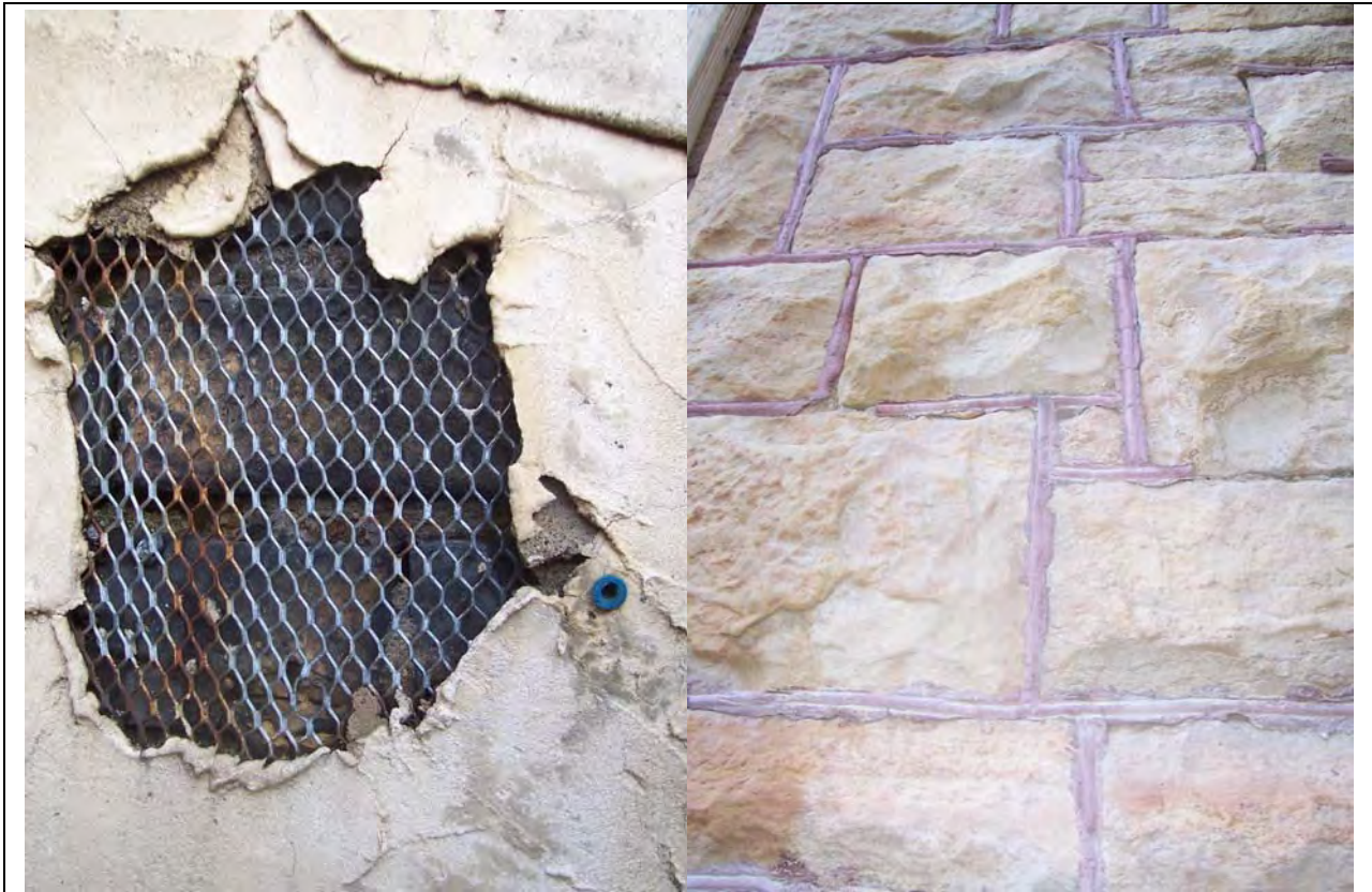
Figure 13. Nonhistoric stucco and maroon mortar, November 2010, source: CPED files
