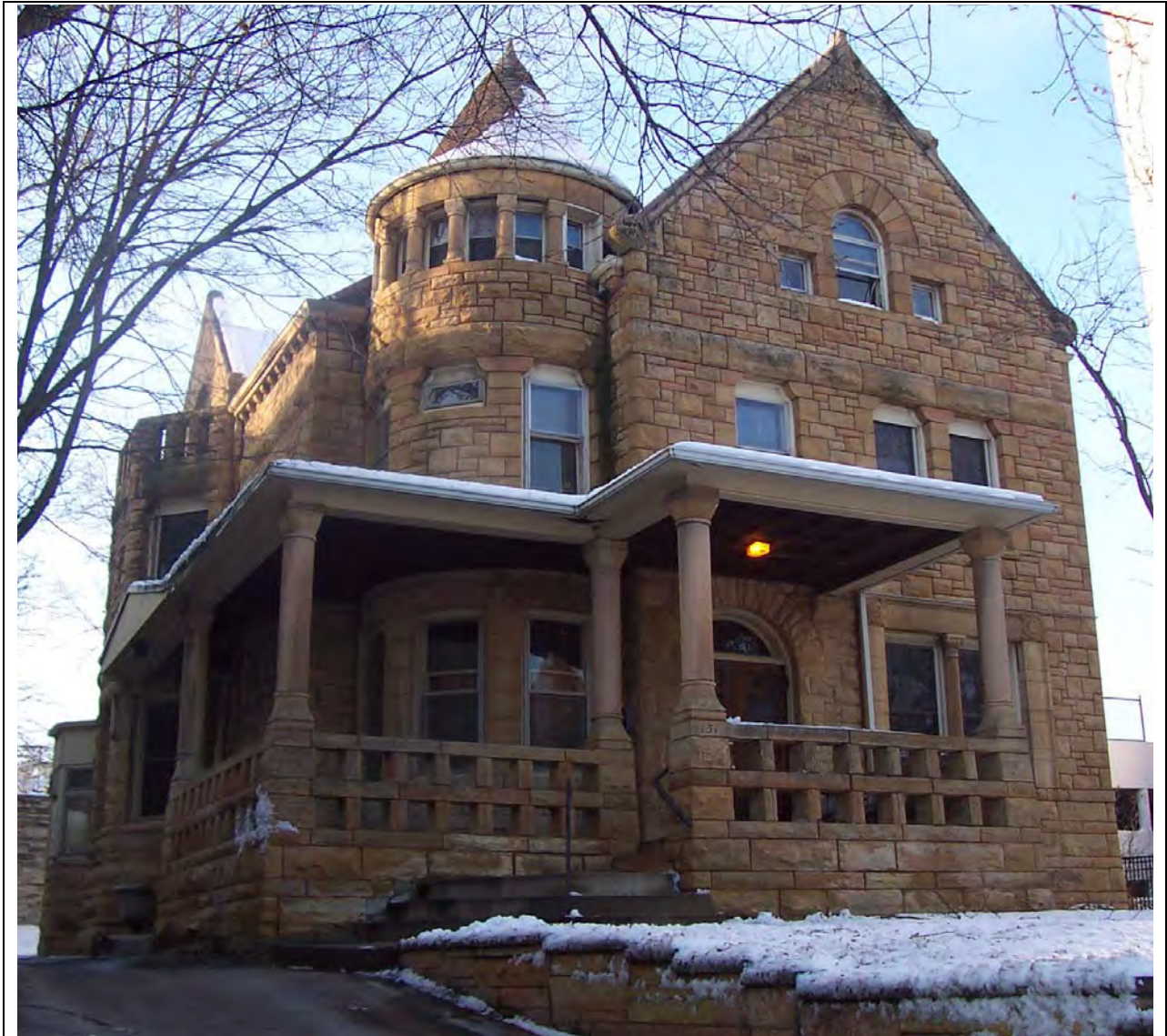
Figure 2. Front (north) elevation and wraparound porch, looking southwest, November 2010, source: CPED files
