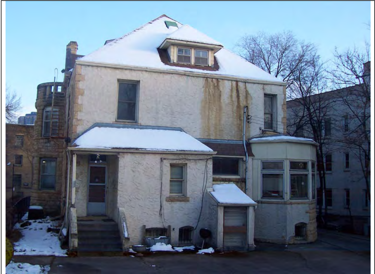
Figure 12. Rear (south) elevation, looking northeast, November 2010, source: CPED files
