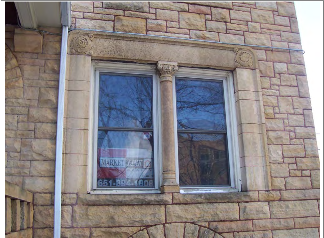
Figure 9. Front windows bearing evidence of columnar porch pattern, looking south, November 2010, source: CPED files
