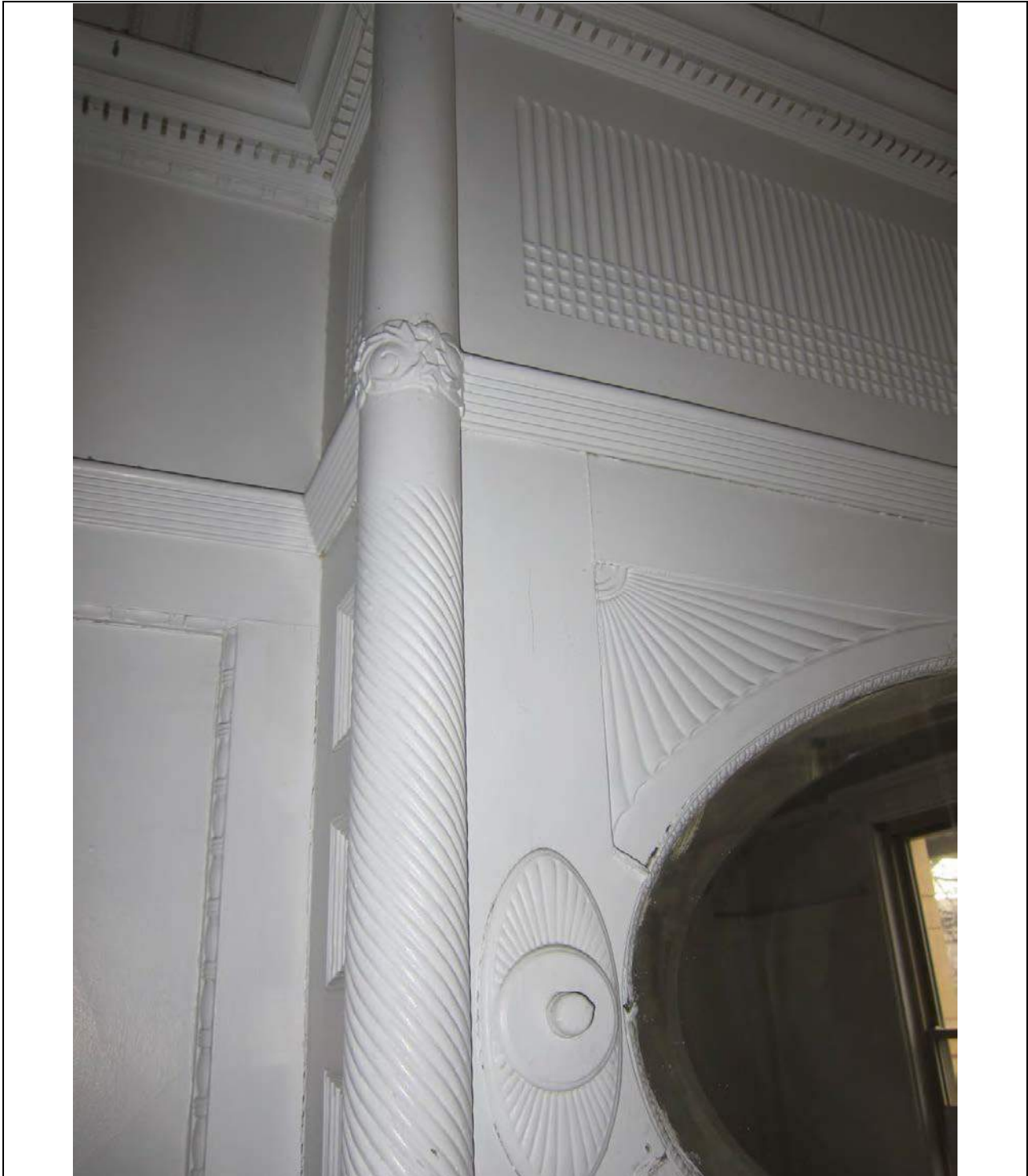
Figure 24. Parlor wall and ceiling details, facing west, November 2010, source: CPED files
