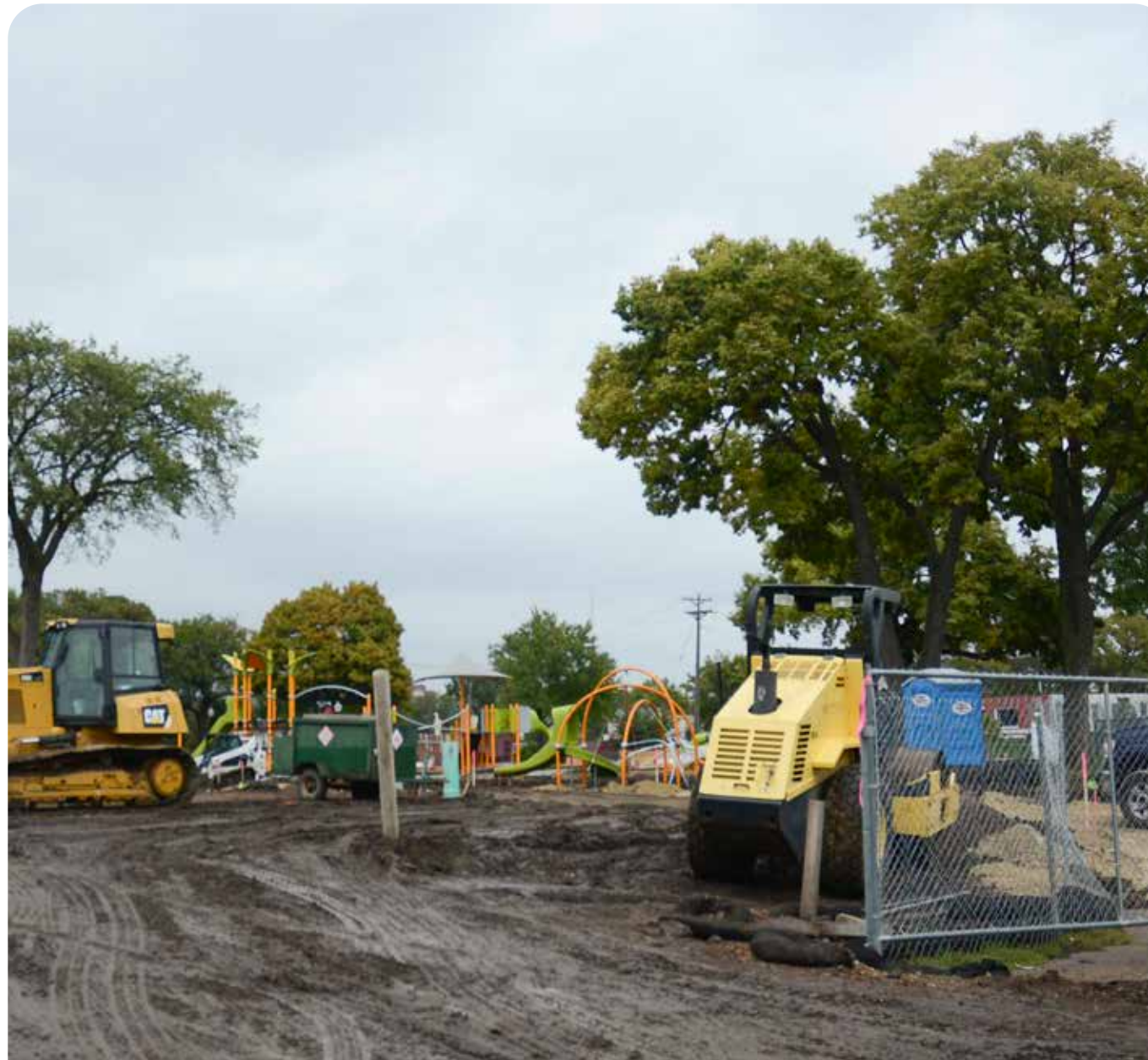
Construction progress at Peavey Park
